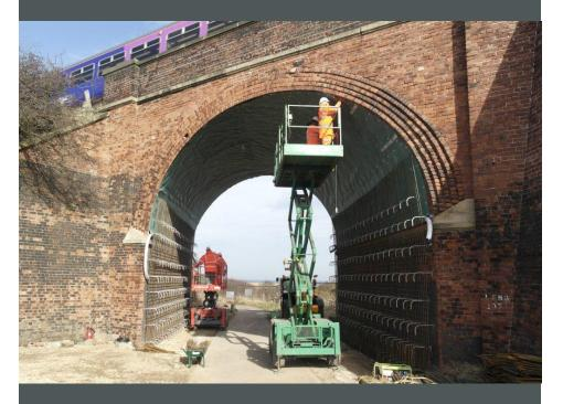
The project required the strengthening of an existing masonry railway arch with a new reinforced concrete liner sprayed insitu. Shotcrete became involved when the Client was looking for alternative methods of construction and Shotcrete worked with Amco and the designers Pell Frischman to alter and optimise the design.
